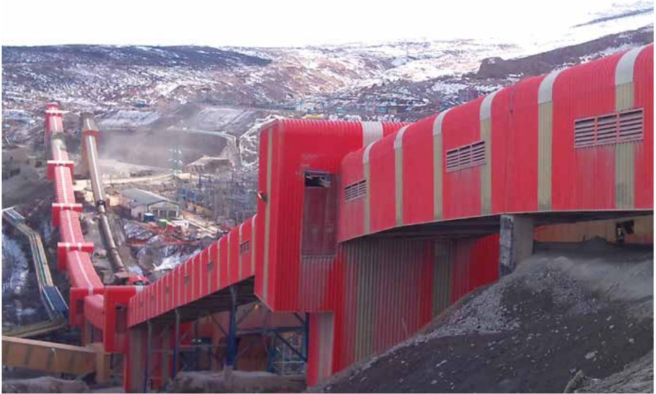
Downhill conveyor for high altitude mining.
